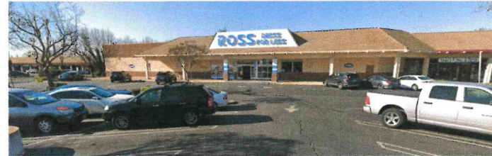
BUILDING C - VIEW FACING WEST
