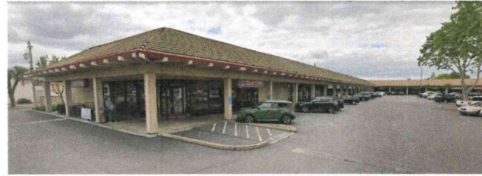
BUILDING A - VIEW FACING SOUTH WEST
