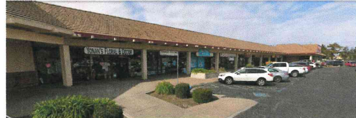
BUILDING D - VIEW FACING NORTH WEST
