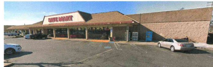
BUILDING D - VIEW FACING SOUTH WEST
