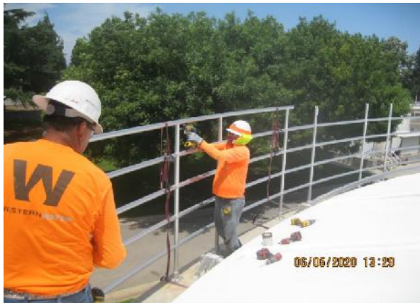
Installation of Digester Guardrail
