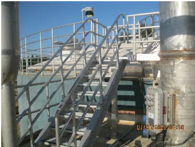
New Staircase for Digester
