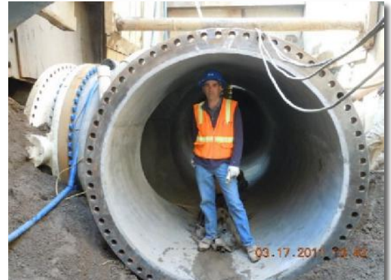
Jeff in 72" Water Transmission Main
