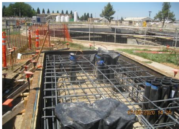
Transformer Pad Ready for Concrete
