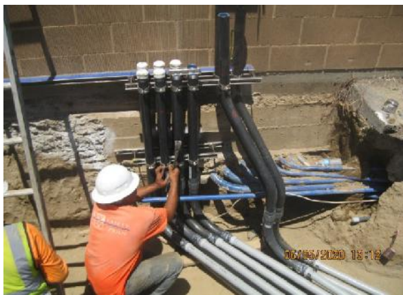
Installation of Screw Press Conduits
