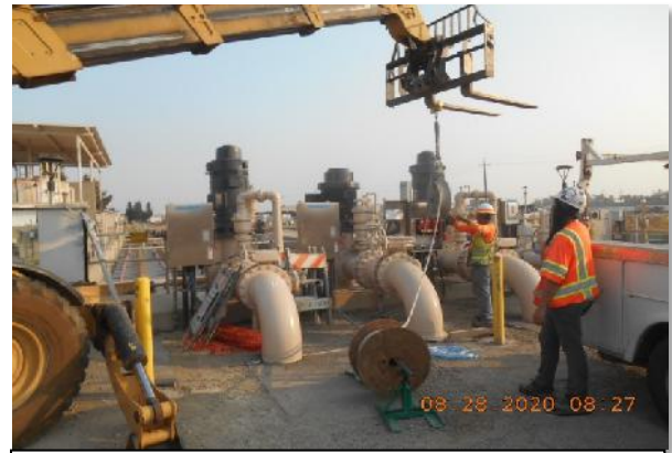
Pulling feeders to Effluent Pumps
