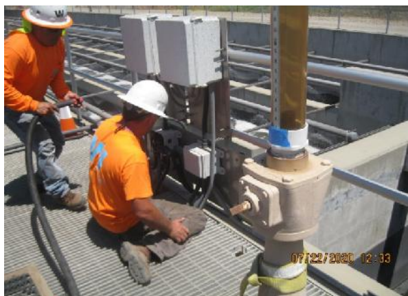
Working on Level Transducers
