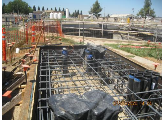
Transformer Pad Ready for Concrete
