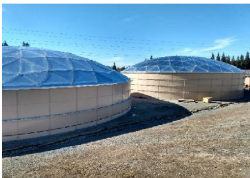
1M Gallon Steel Bolted Tanks
