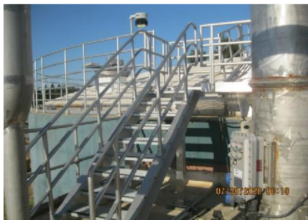
New Staircase for Digester
