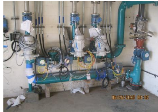
Wiring Motor Operated Valves on 6" DS
