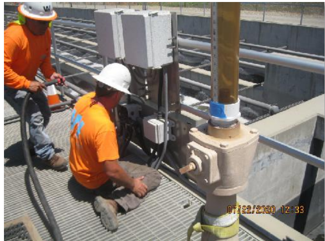
Working on Level Transducers
