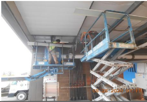
Dewatering Canopy Lighting and Soffit
