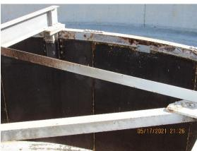
The feed well and supporting structural steel is exhibiting isolated corrosion that can lead to pitting due to metal loss.
