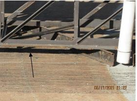
The rake arms are exhibiting edge corrosion on about 10% of the structural steel. This is active isolated corrosion that will cause metal loss. The scraper blades on the bottom has active corrosion.
