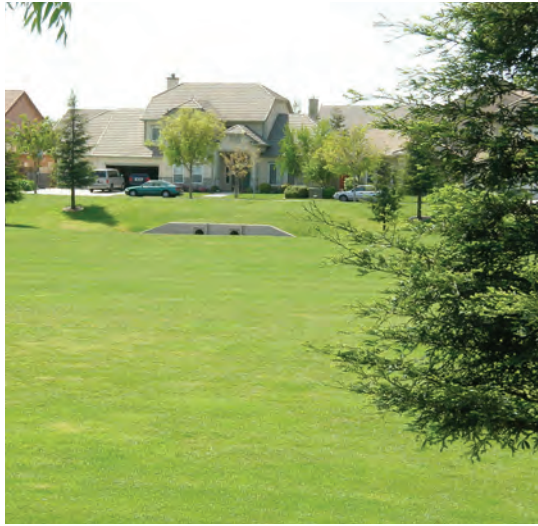
Detention basins are distributed throughout the City, capturing runoff during stormwater events. Some of these detention basins also serve as City parks.
