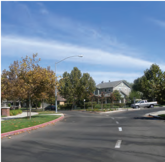
Characteristics of many newer neighborhoods in Turlock include front-accessed garages, cul-de-sacs, and curvilinear street systems.
