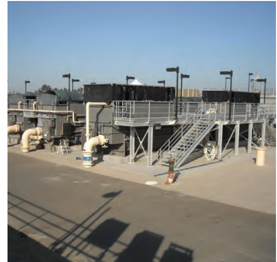
Tertiary Filters at the RWQCF help treat the water to a very high level, allowing it to be used in the community for landscape irrigation, for agricultural irrigation, for cooling water, or other nonpotable uses.
