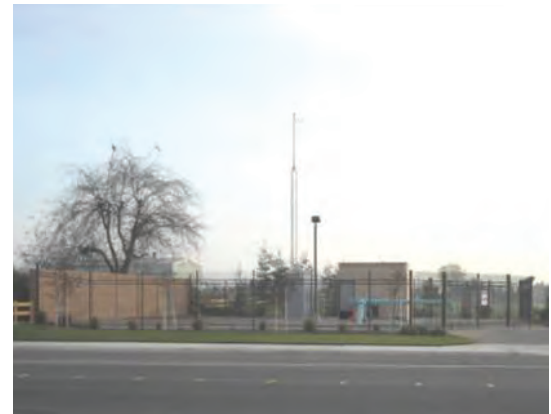
Turlock's potable water supply comes entirely from groundwater. One of the city's newest wells was constructed in 2007 near the northeast greenbelt.
