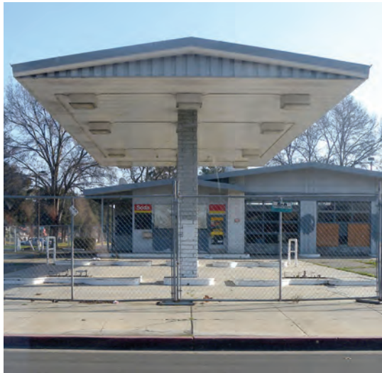
Railroad lines and storage of chemicals present potential hazards in the Study Area (top).
