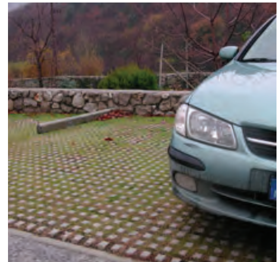
Permeable paving materials help manage stormwater runoff by allowing water to filter into the ground on site.
