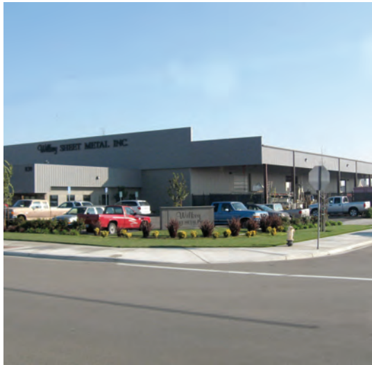
The adoption of the Westside Industrial Specific Plan has enabled substantial new industrial development on large parcels west of Highway 99.
