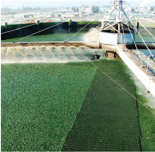
The RWQCF, last upgraded in 2006, treats wastewater from Turlock and the neighboring communities of Keyes and Denair.
