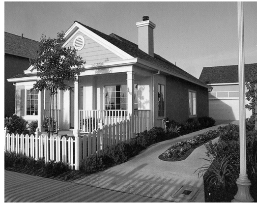
Example of a garage located at the rear of the lot behind the dwelling.
